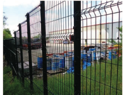
Industrial Works along the A64
