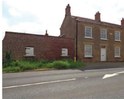
Manor Farm and wall along the A64
