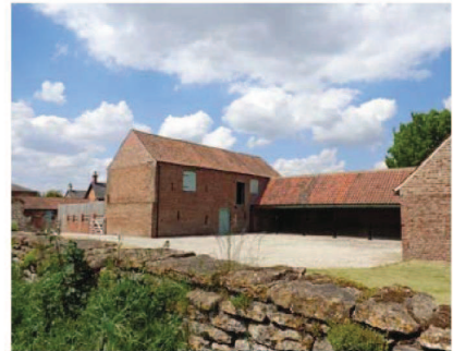
Traditional dwelling - Corner House Farm (Listed Building)
