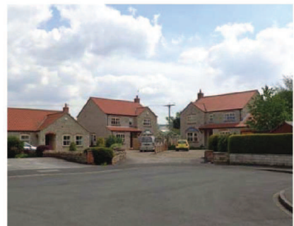
Modern housing along Eastbeck Close
