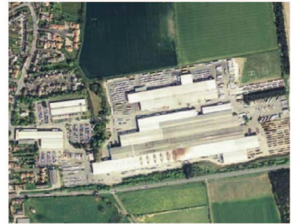
Industrial Warehouses (Kingspan and Atlas Ward Structures)
