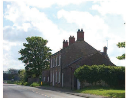
T13 Sycamore along the A64
